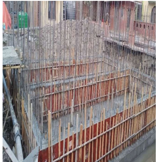
Under construction of semi underground reservoir at Indrakamal pump house, Lokanthali
