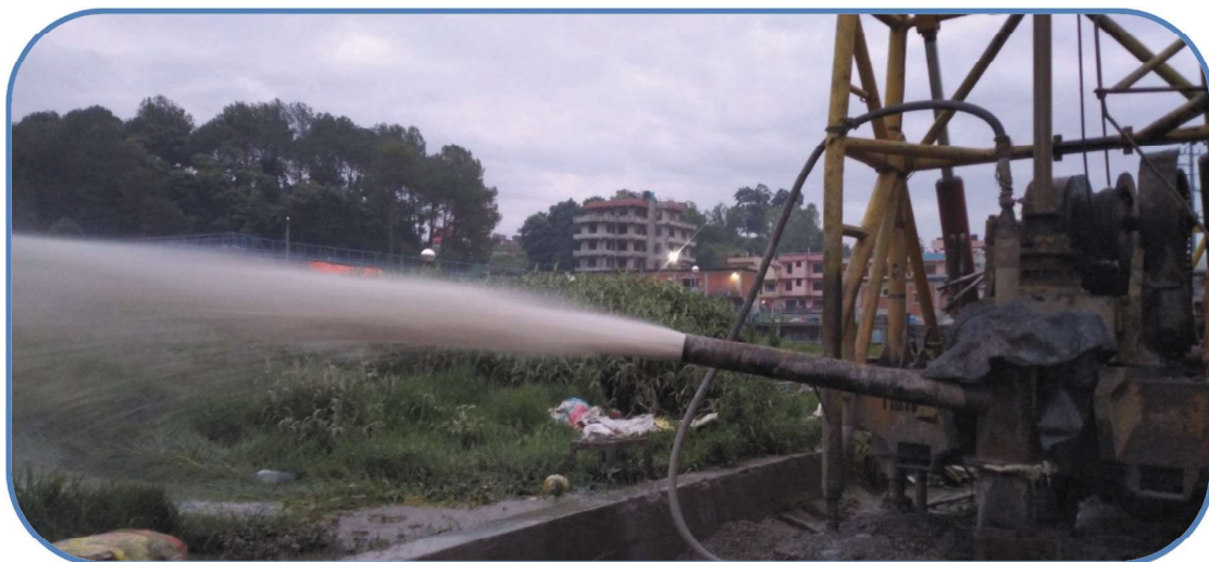
New Tubewell Drilling Works
