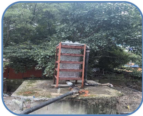
Aeration and Sedimentation Tank at Ratnapark WTP
