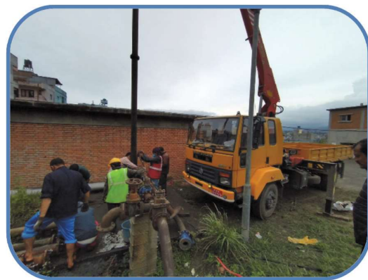
Pump Replacement in Tubewells
