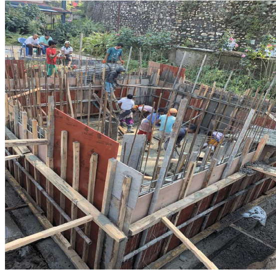
Semi underground reservoir at Gokarneshwor
