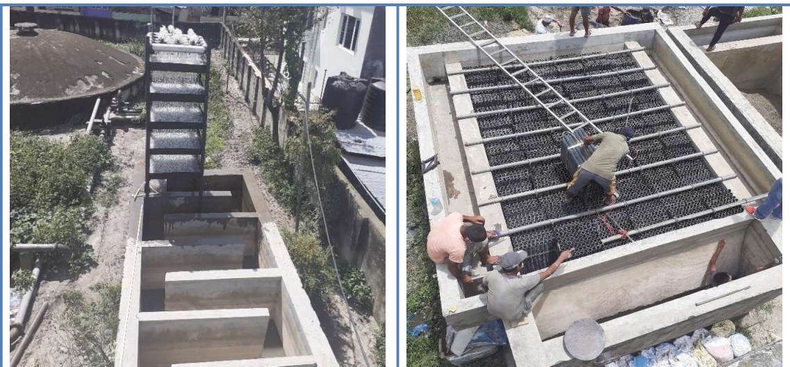
Flocculation and Aeration Unit
