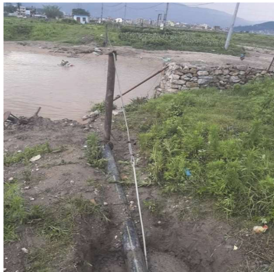
Intake pipeline maintenance at Manohara River
