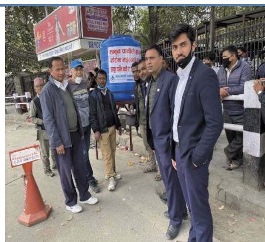
Final Installation of Hand Wash Station
