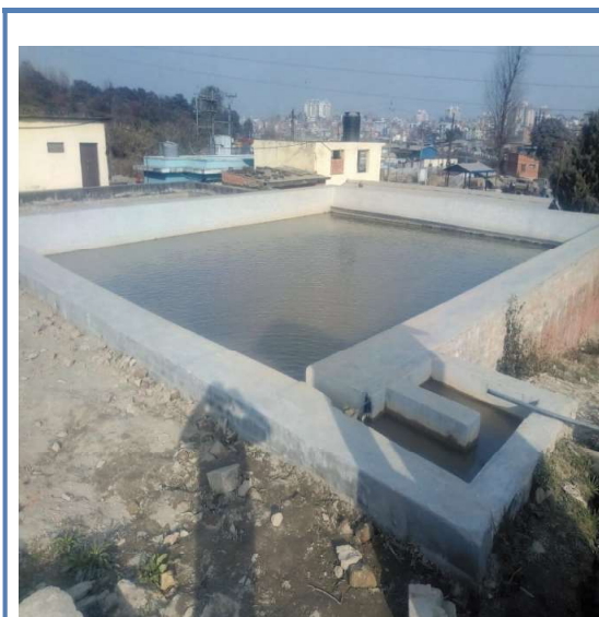
Conversion of Slow Sand filter to Sedimentation Tank
