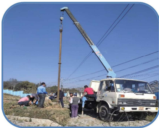
Pump Replacement in Tubewells
