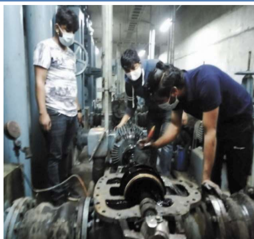
Horizontal Split Centrifugal Pump Repair
