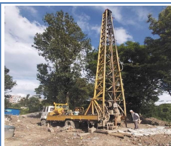
Drilling of New Deep Tubewell
