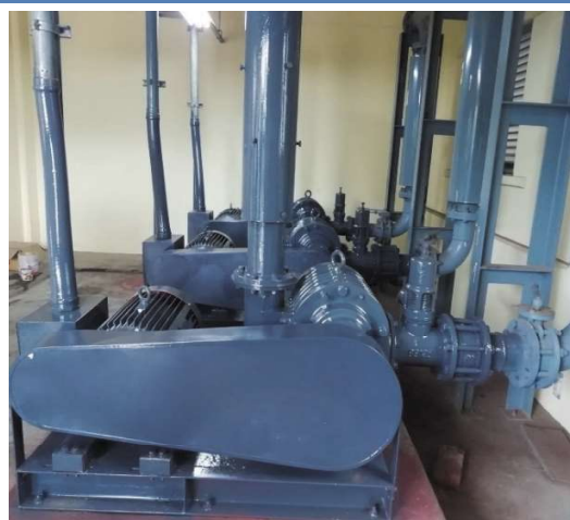
Blower/Compressor Repair Works
