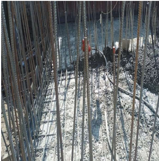
Base concreting of Rapid sand filter at Lokanthali treatment plant
